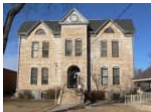
Greeley County old courthouse from south
